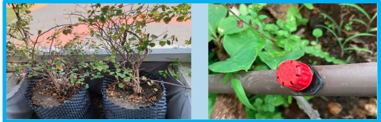
The drip irrigation system
